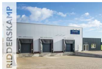
Warehouse and Service Centre
